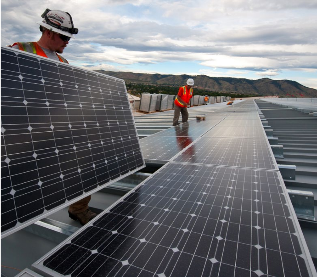
Workers install solar panels in the U.S. ©U.S. Department of Energy/Schroeder.
